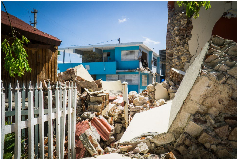
Figure 2: Damage from 6.4 earthquake on January 7, 2020 in Guayanilla
